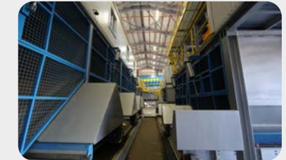
13 AUTOMATIC BUNKER SYSTEM
