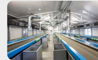
10 QUALITY CONTROL CABIN
